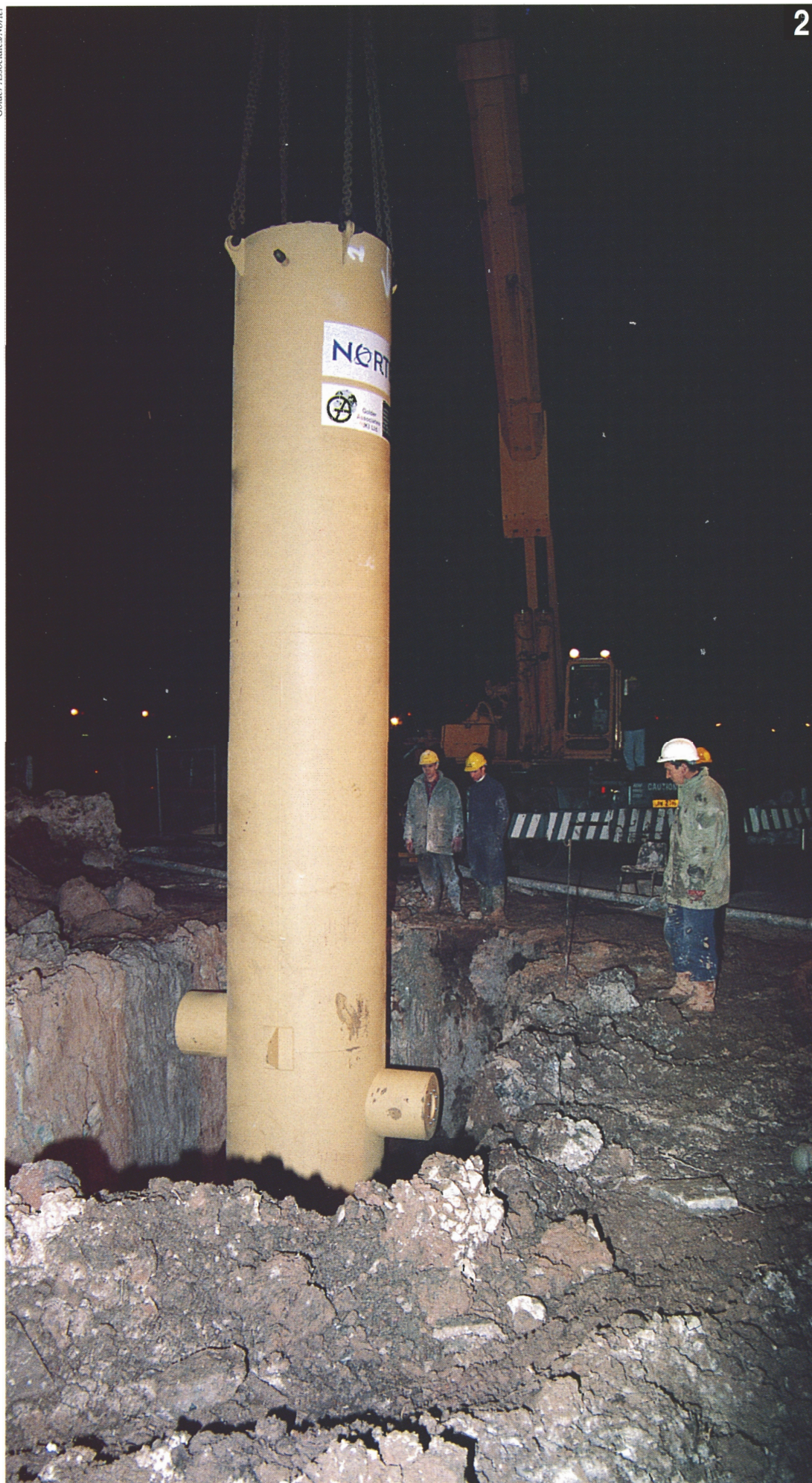
Installation of the reactor vessel 'gate' contained within a cement bentonite slurry wall 'funnel', which is successfully treating a localised plume of TCE at Nortel's site in Belfast
